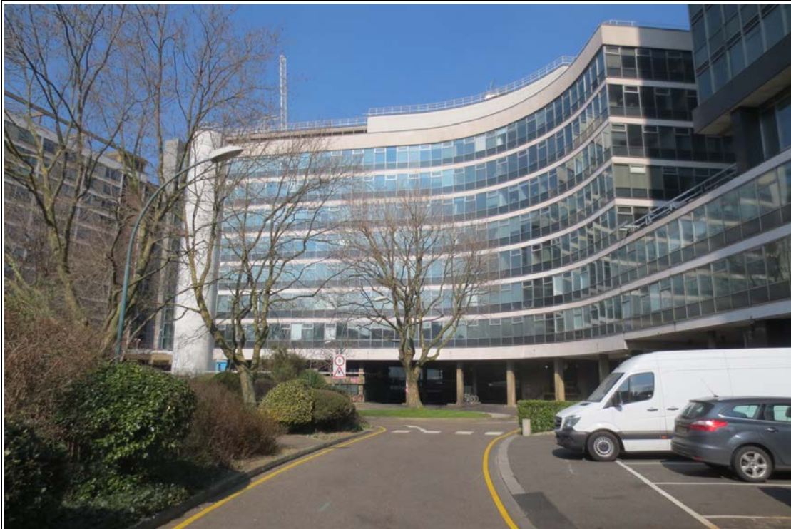
View of rear of 'Y' Building
