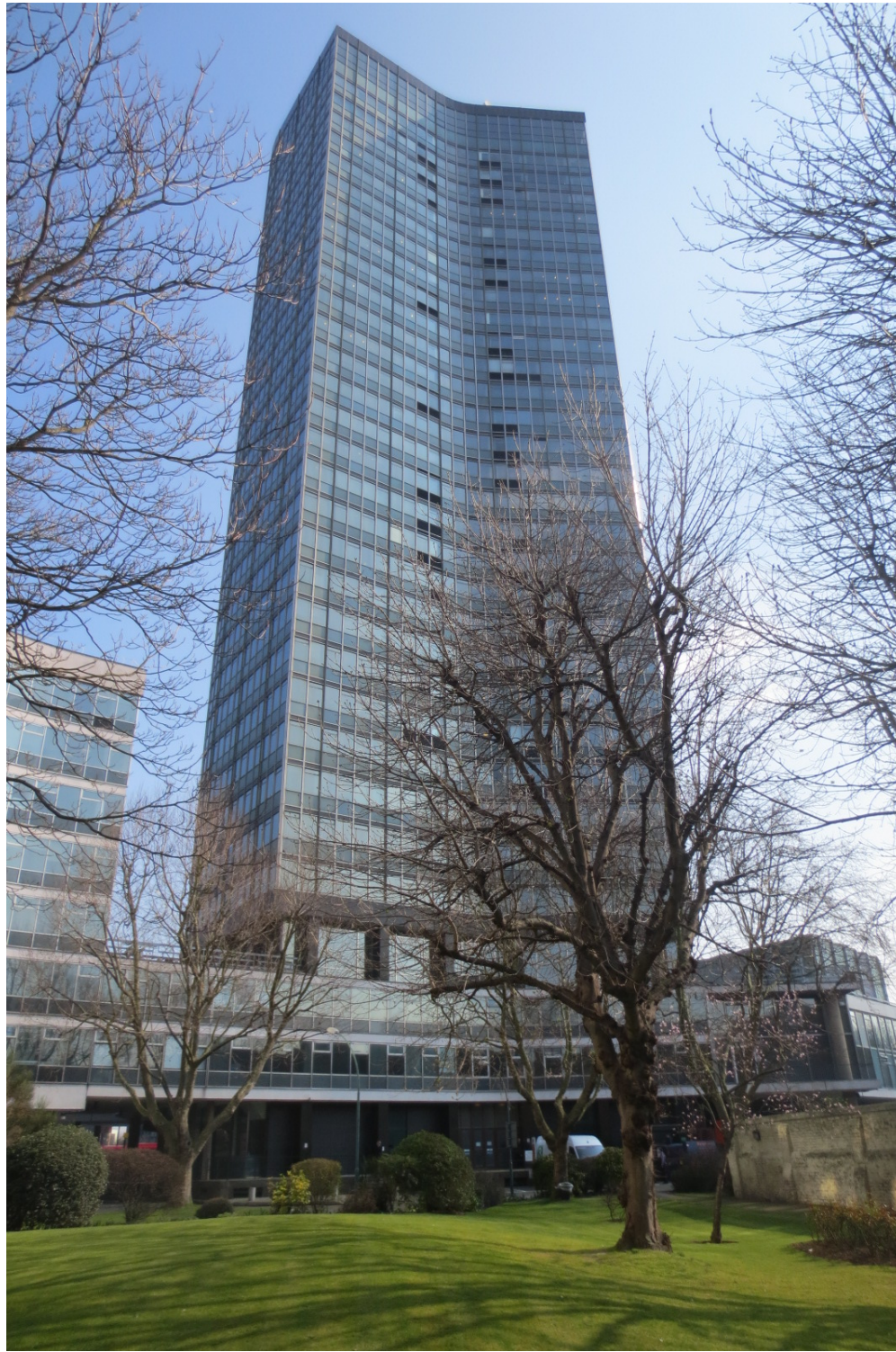
View of Tower from rear gardens
